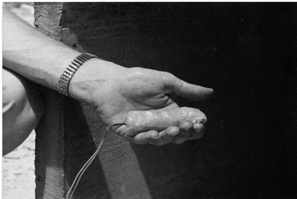
Figure 20. A \frac{1}{4} pound charge of Composition C-3 explosive.
