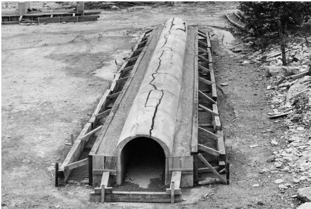
Figure 59. The damage resulting from the demolition applied to the tunnel in Test Two, Phase V.
