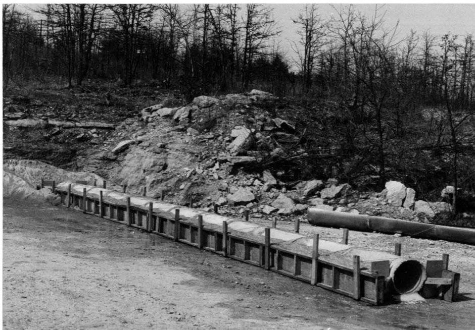
Figure 61. The Type C tunnel constructed for Test Two, Phase VII.
