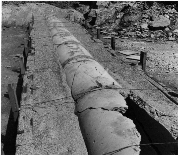
Figure 63. The results of demolition Test Two, Phase VII.
