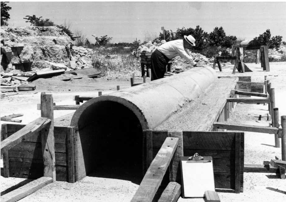
Figure 30. Type A tunnel constructed for Test Four, Phase II.
