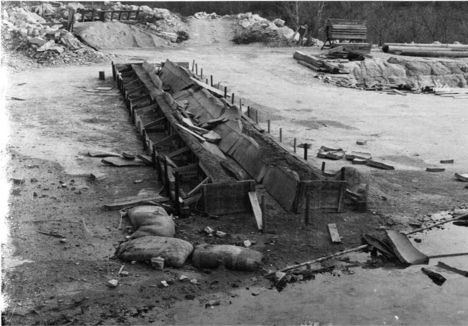
Figure 56. The Phase IV tunnel after demolition.
