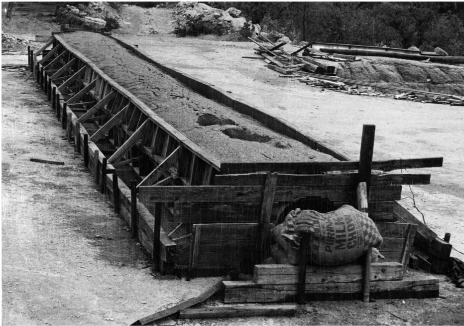
Figure 52. The results of demolition in Test Five, Phase III.
