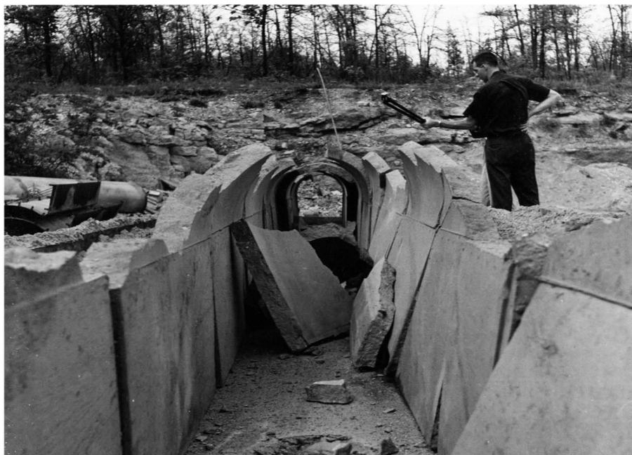
Figure 60. The results of demolition in Phase VI.
