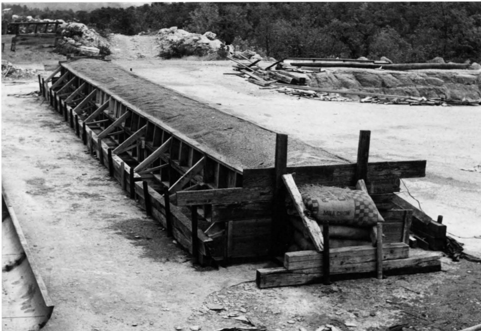
Figure 51. Sand bags approximately 18 inches thick closed the portal in Test Five, Phase III.
