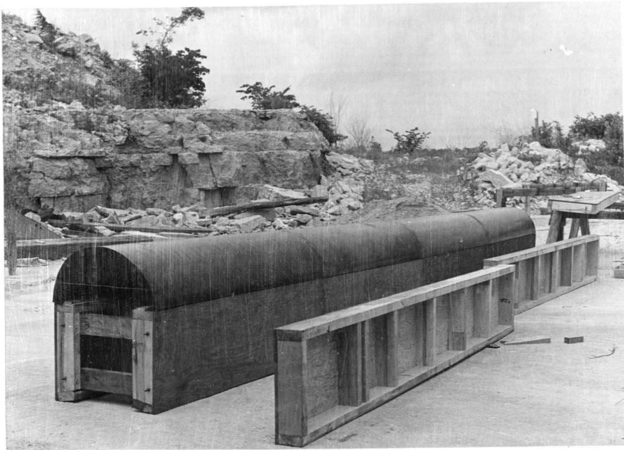
Figure 3. Inside metal arch forms.
