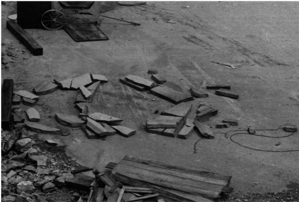
Figure 23. The results of demolition in Test Two, Phase One.
