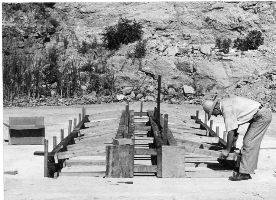
Figure 2. Wooden forms held in position with braces
