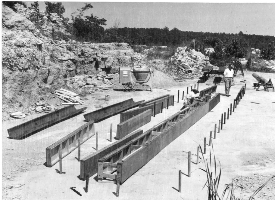
Figure 1. Lag bolts were used to join wooden forms
