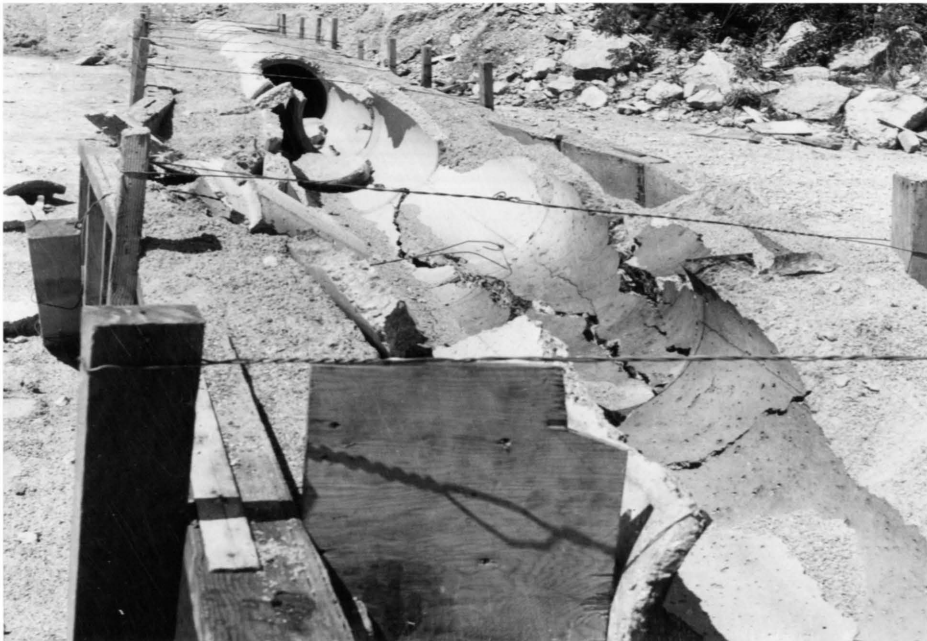
Figure 69. The results of demolition in Test Three, Phase IX.
