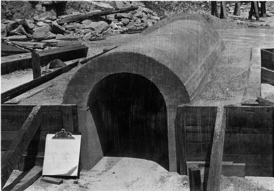
Figure 28. Type A tunnel constructed for Test Three, Phase II.
