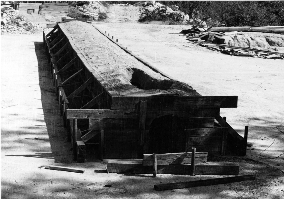
Figure 49. The results of demolition in Test Four, Phase III.
