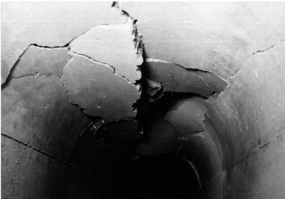
Figure 53. The results of demolition in Test Five, Phase III.
