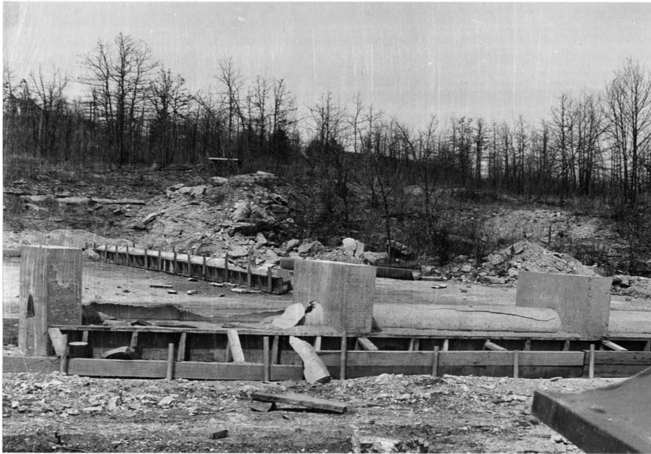
Figure 46. The results of the demolition in Test Eight, Phase II.
