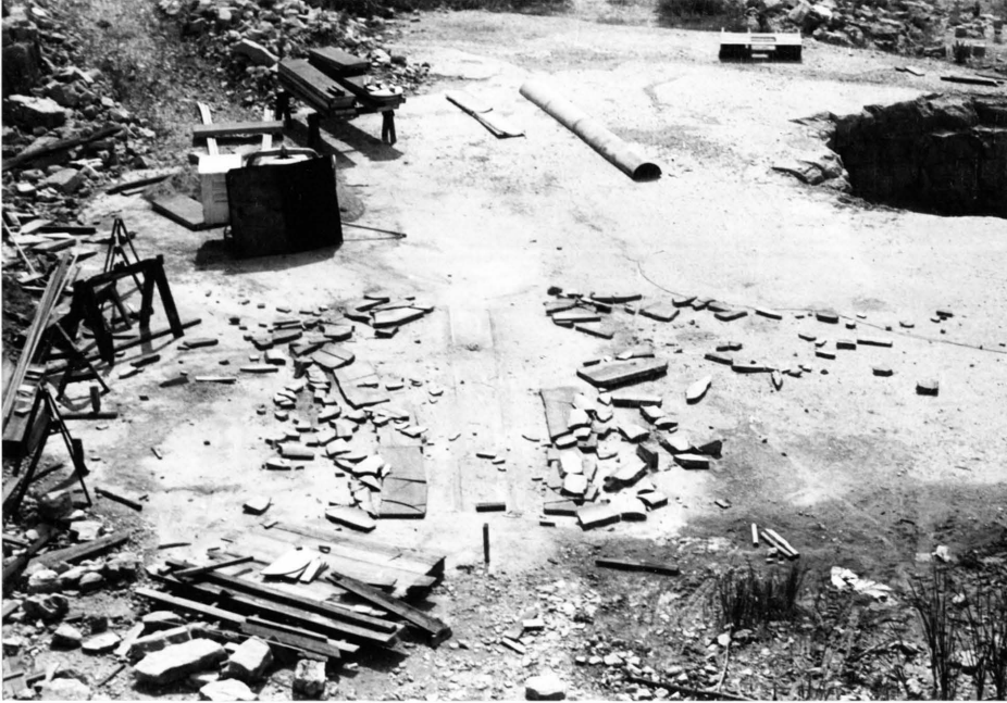
Figure 27. The results of demolition in Test Two, Phase II
