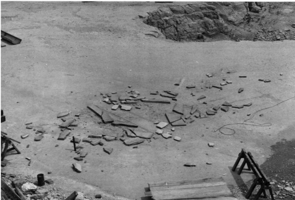
Figure 21. The results of demolition in Test One, Phase One.
