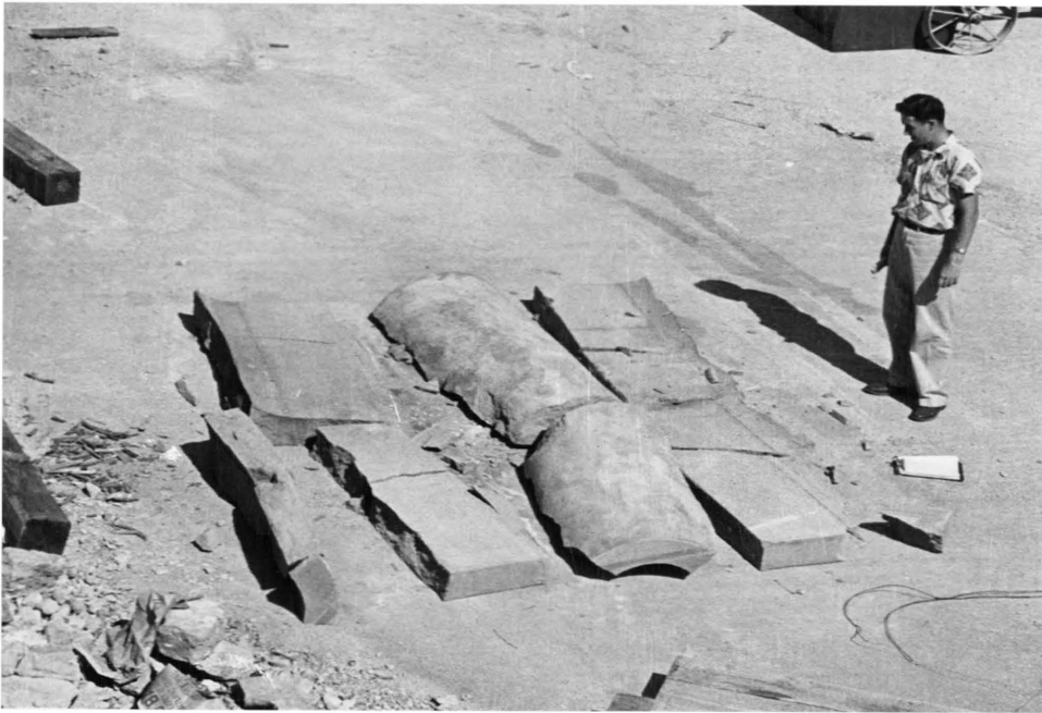
Figure 25. The results of demolition in Test Three, Phase One
