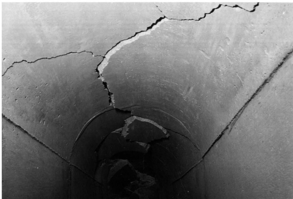
Figure 48. The results of demolition in Test Two, Phase III.
